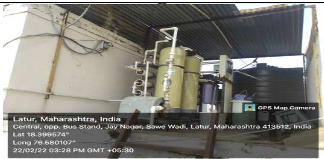
RO Plant on the Roof in Main Campus
