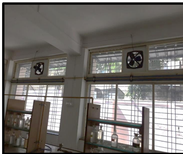
Exhaust fan in laboratories for ventilation
