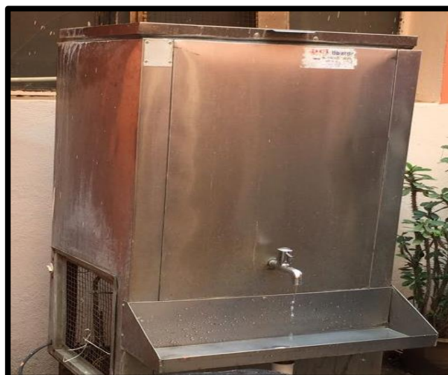
Leaking tap in main campus building
